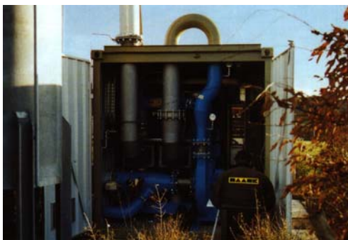
View inside the VocsiBox®-container IN BARSBÜTTEL
